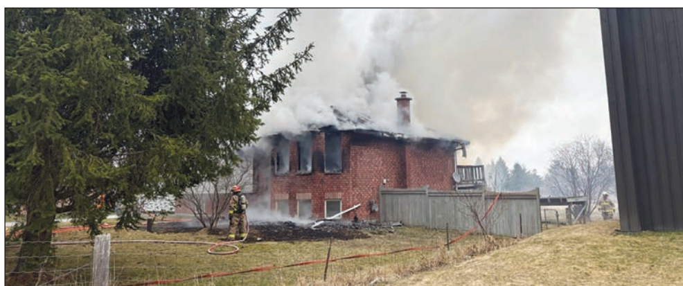
TRAGIC BLAZE – A fire at a property in Essa claimed one person's life on April 15. The fire has been deemed non-suspicious and no foul play is suspected in the death of the individual. BRIAN LOCKHART PHOTO
